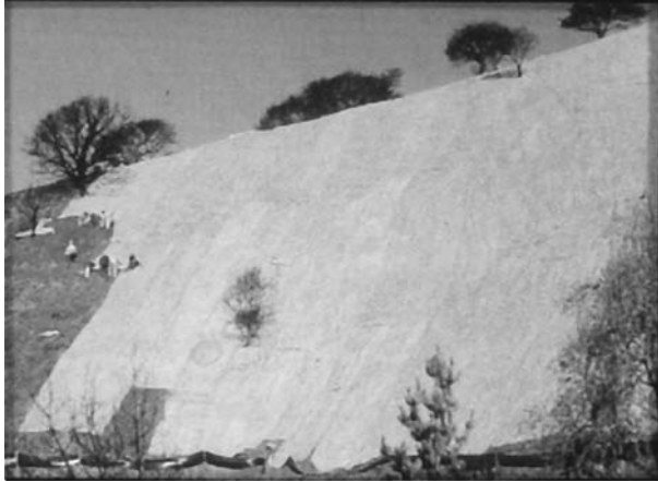
FIGURE 7.10 Geotextile used to stabilize a steep slope (USDA).
